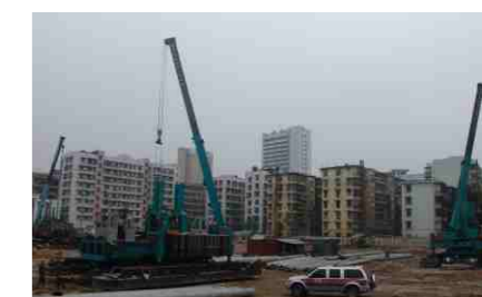
天津施工 Construction scene in Tianjin
