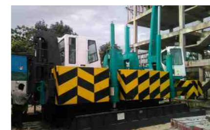
缅甸施工 Construction scene in Burma
