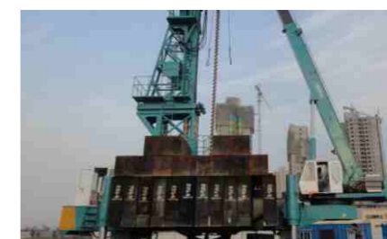
河南施工 Construction scene in Henan
