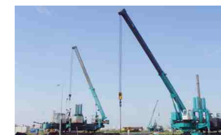
越南施工 Construction scene in Vietnam
