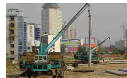
武汉施工 Construction scene in Wuhan
