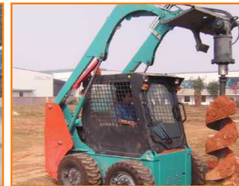
Construction in Changsha
